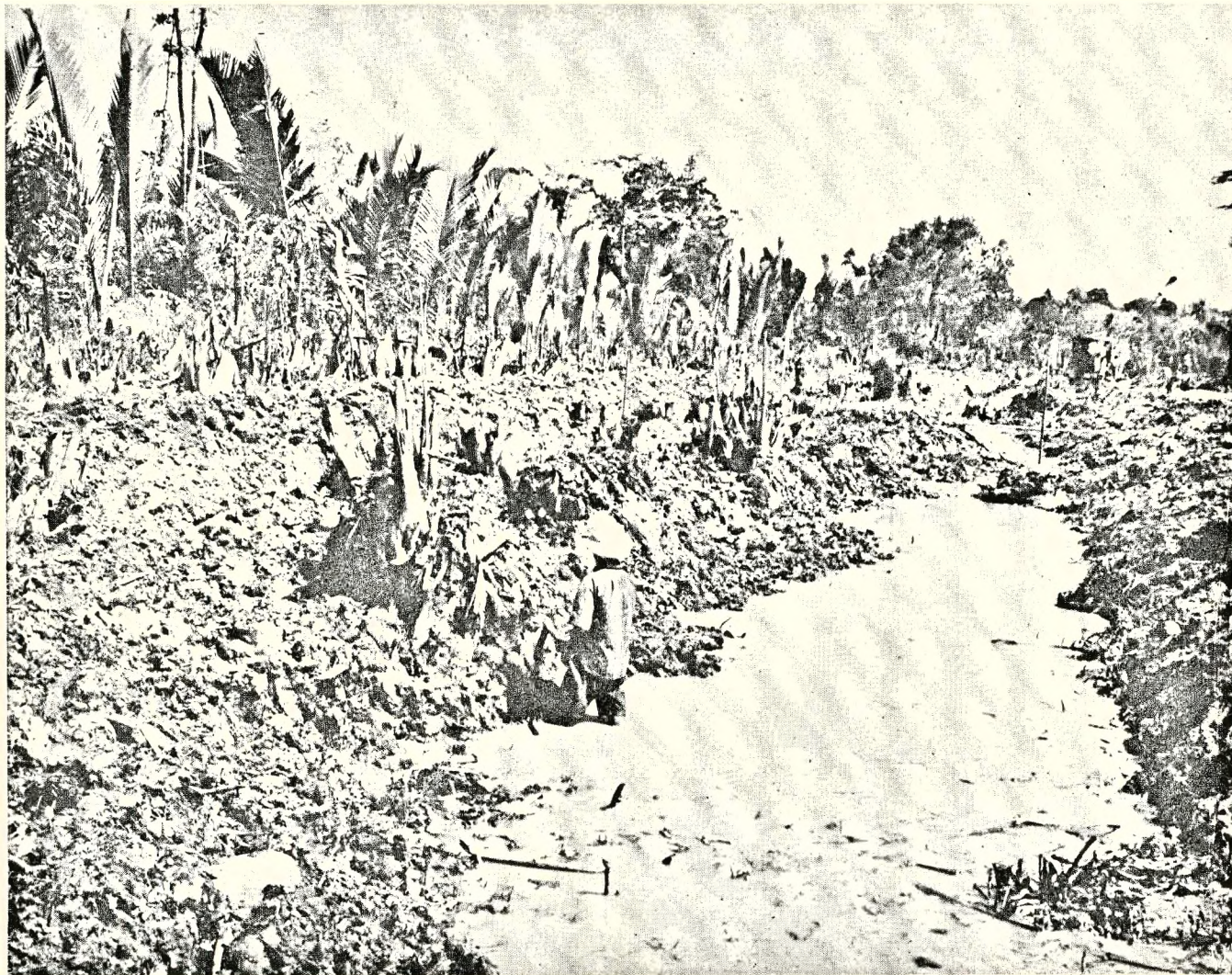
CONNAUGHT BRIDGE POWER STATION. Excavating the circulating water outlet pipe trenches through Swamp.
