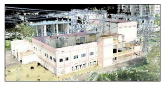
Fig. 2 Scanning of PMU Seberang Jaya using TLS
