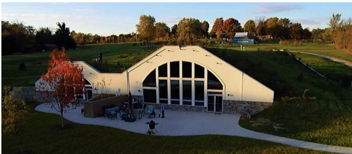
Fig. 2. An example of the ground Bermmed house. Reproduced from <https://homedesignfree.com/berm-home-designs.html/>
