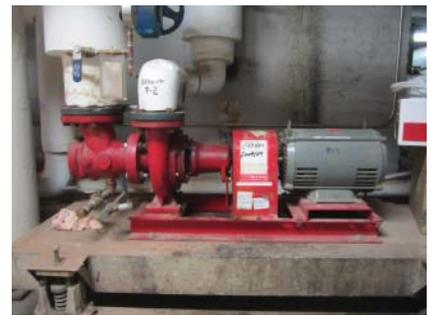
**Figure 8.33** Base-mounted pump.
