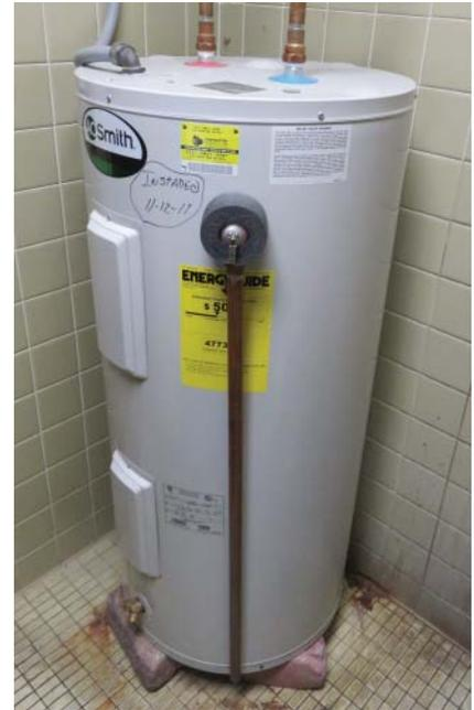
Figure 12.5 Electric water heater.
