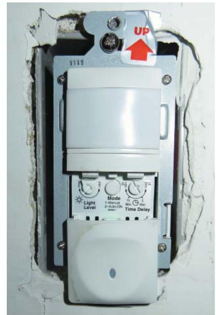
Figure 5.26 Control settings inside a wall-mounted vacancy sensor.
