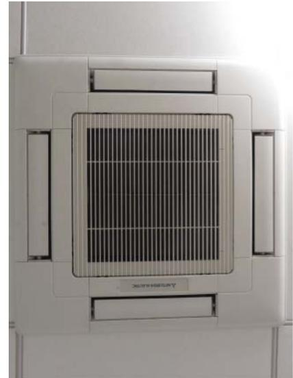
**Figure 7.15** Ceiling-recessed ductless indoor unit (cassette).
