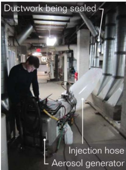
**Figure 8.16** Aerosol duct sealing.
