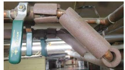
Figure 8.27 Inadequately insulated piping—inadequate insulation thickness, elbows and fittings not insulated, insulation does not fully cover piping, sections of piping are not insulated.
