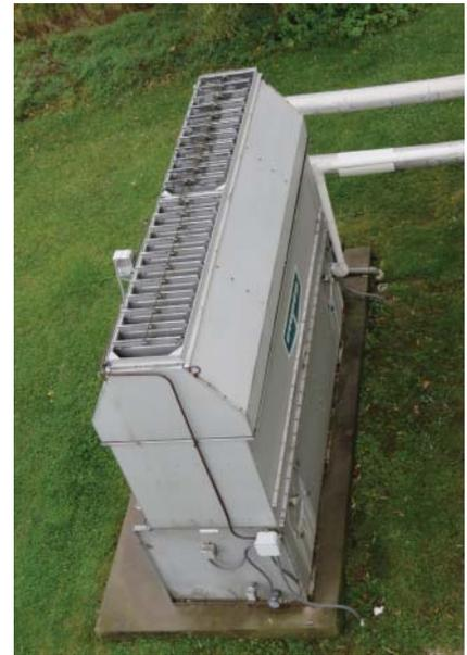
**Figure 7.36** Ground-mounted cooling tower.
