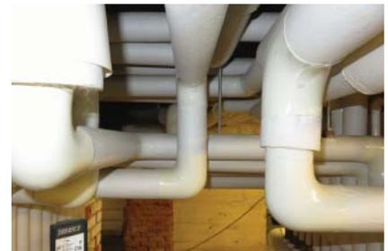
Figure 8.26 Professionally insulated piping—adequate insulation thickness, elbows and fittings insulated, no piping missed.
