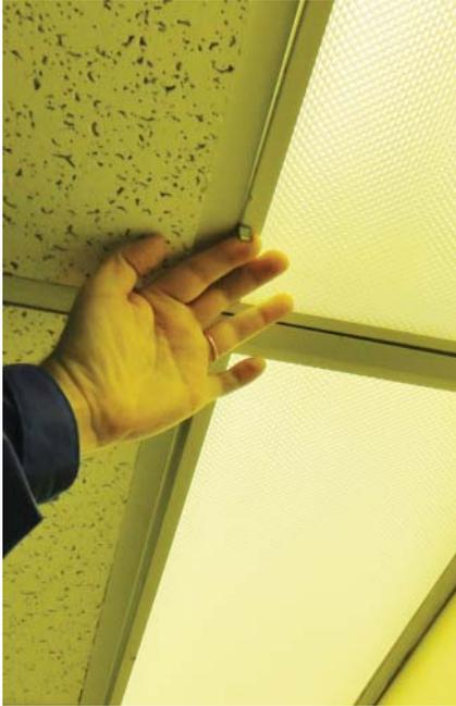
Figure 5.15 Opening a troffer fixture.
