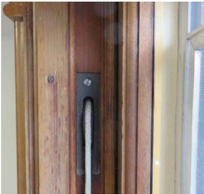
**Figure 4.10** Double-hung window sash counterweight.
