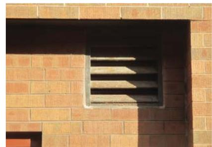
**Figure 9.12** Louvers serving an outside air intake.
