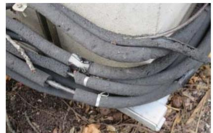
**Figure 8.39** Deteriorated exterior refrigerant pipe. insulation
