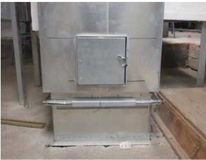
Figure 8.10 Duct access panel.
