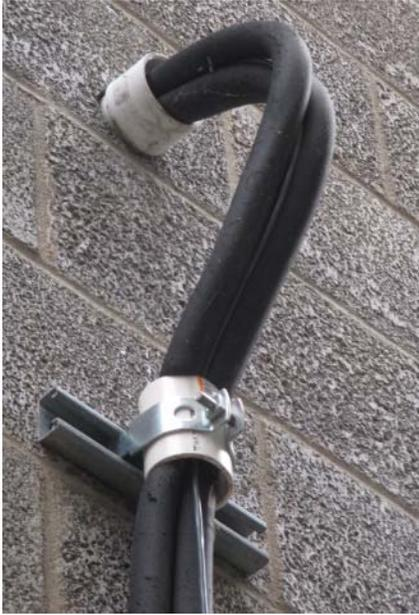
**Figure 4.58** Air conditioner piping penetrating an exterior wall.
