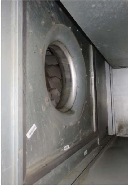
Figure 8.21 Centrifugal fan.
