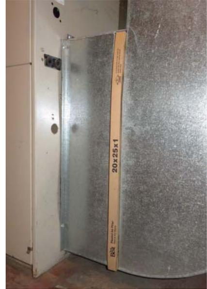
**Figure 8.7** Leakage at duct connection to furnace and at filter housing.
