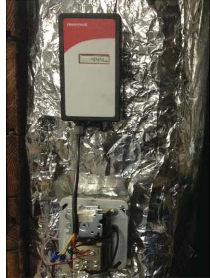
**Figure 9.15** Carbon dioxide control mounted on return duct.
