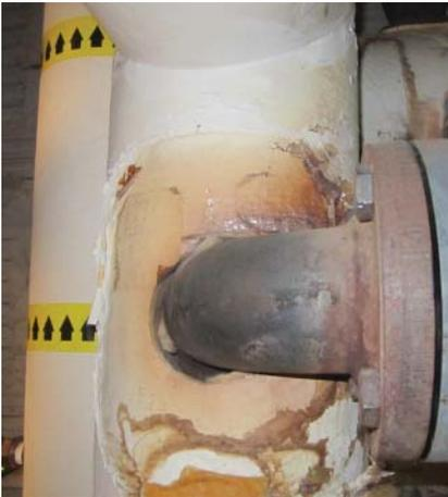
Figure 8.29 Uninsulated flanged elbow.
