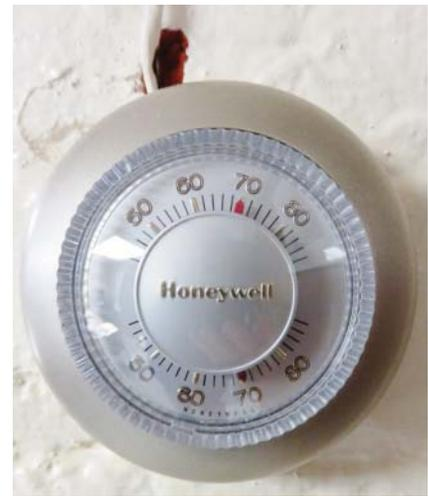
Figure 11.5 T86 wall-mounted thermostat.
