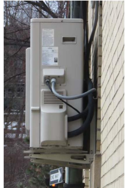
**Figure 7.19** Heat pump outdoor unit mounted too close to a wall.
