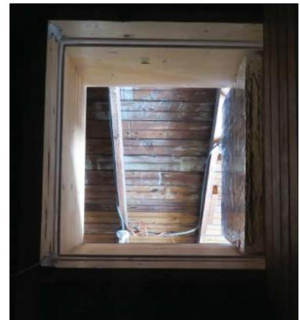
**Figure 4.18** Attic hatch with dam to prevent cellulose spilling into hatch.
