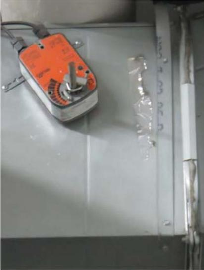
**Figure 11.16** Duct damper motor actuator.
