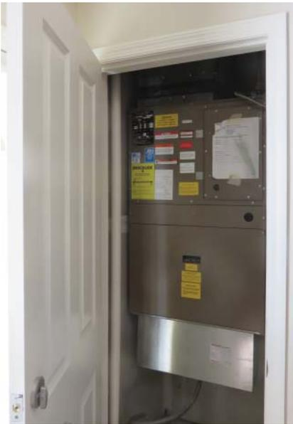
**Figure 7.28** Indoor through-wall single-package unit.
