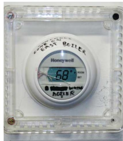
Figure 11.9 Thermostat inside cover.
