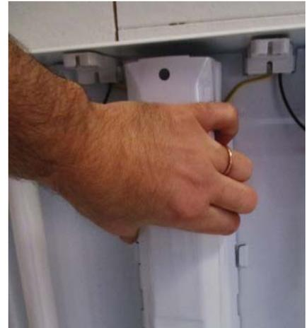
Figure 5.4 Removing sheet metal cover to access a fluorescent fixture ballast.
