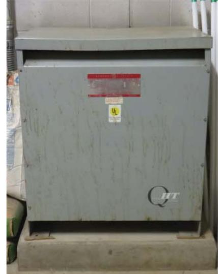
Figure 13.4 75-kVA transformer.
