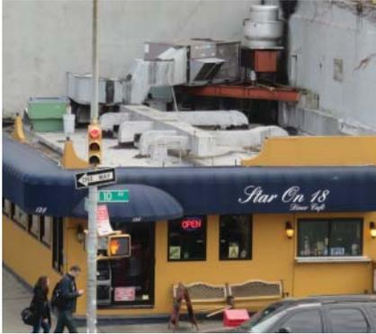
**Figure 10.3** Rooftop equipment—note upblast exhaust fan, an indicator of a commercial kitchen; also heating and cooling rooftop unit with outdoor supply ductwork, and outdoor air intake.
