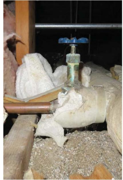
**Figure 8.32** Asbestos insulation on water pipe.
