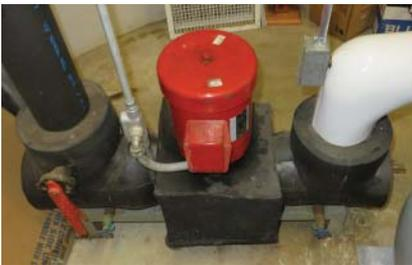
Figure 8.30 Insulated valve (left), pump body (center), and elbow (right).
