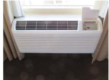
**Figure 7.4** Packaged terminal air conditioner (PTAC).
