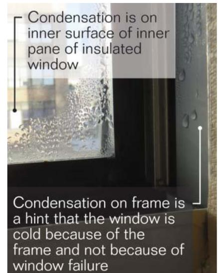
Figure 4.46 Window condensation.
