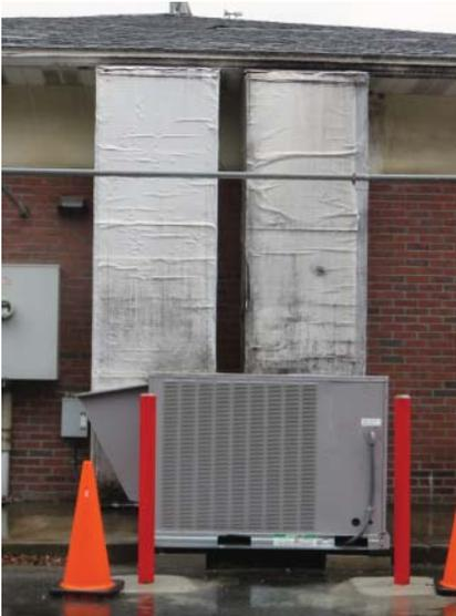
Figure 7.22 Ground-mounted single-package unit
