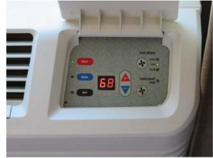
Figure 11.4 Equipment-mounted electronic thermostat.
