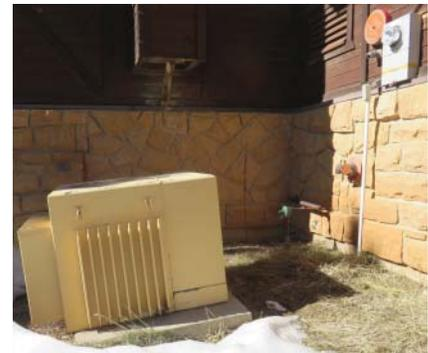
Figure 13.5 Pad-mounted transformer—the electric meter (top right) is an indication that this transformer is on the utility side of the meter.
