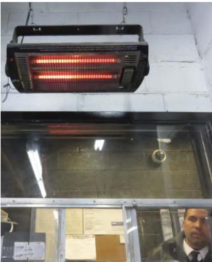
Figure 6.25 Electric infrared heater.
