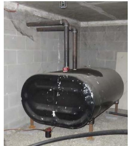
Figure 6.1 Heating fuel oil tank.
