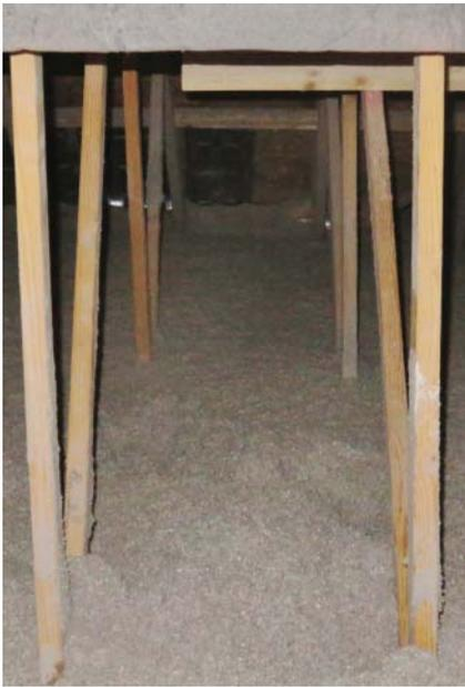
**Figure 4.16** Cellulose insulation in attic.
