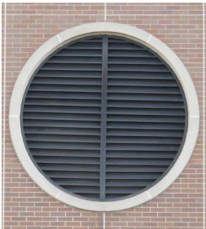
**Figure 10.4** Ventilation outdoor air intake.
