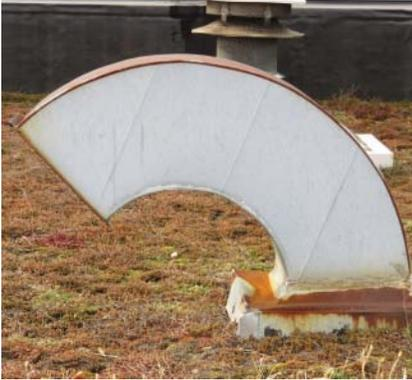
**Figure 9.7** Gooseneck air intake on a vegetated roof.
