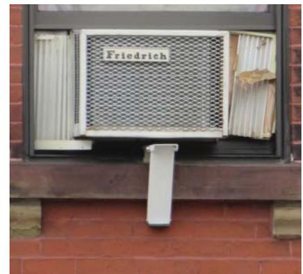
**Figure 4.65** Room air conditioner with leakage around window mounting.
