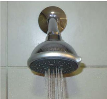
Figure 12.21 Showerhead, 2.1 GPM.
