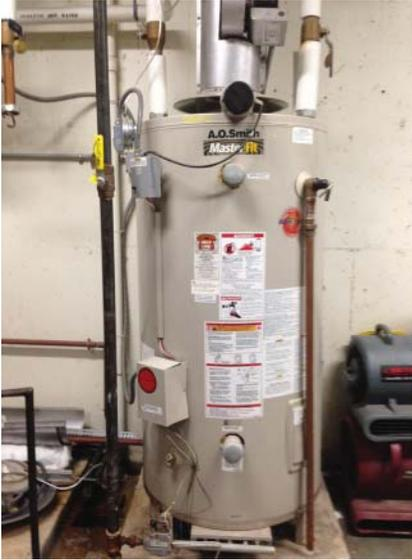
**Figure 12.3** Natural gas commercial storage water heater.
