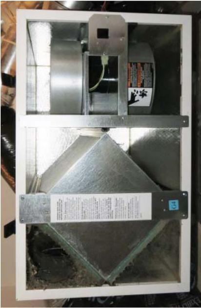
**Figure 9.19** Flat plate recovery ventilator—heat exchanger is at the bottom, supply and exhaust fans are at the top.
