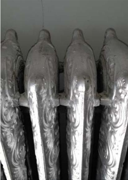
**Figure 6.14** Cast iron steam radiator without pipe connection across the top—cannot be converted to hot water.
