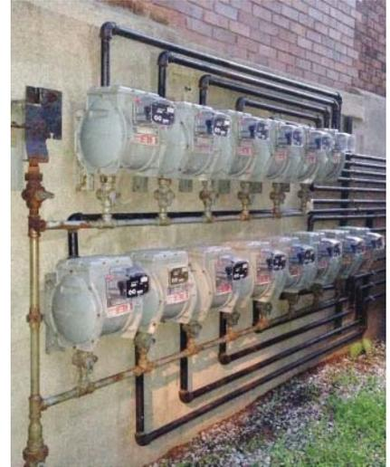
**Figure 21.3** Energy managers should take their own meter readings, to increase the frequency of readings, for purposes of energy diagnostics.
