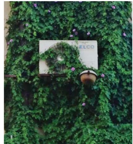
**Figure 7.20** Vegetation covering a heat pump outdoor unit.
