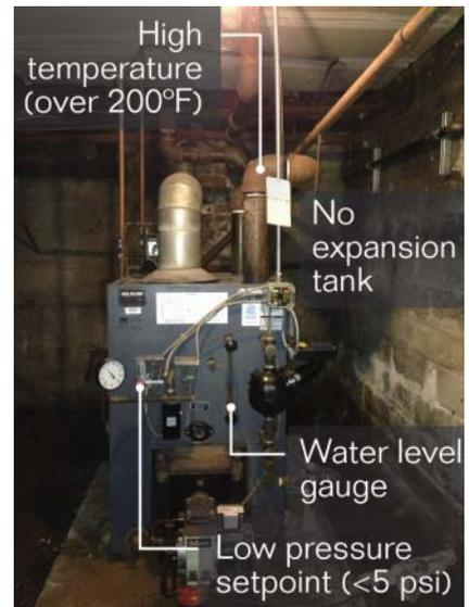
Figure 6.10 How to identify a steam boiler.
