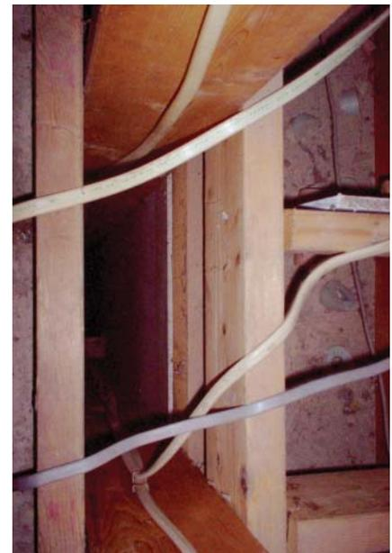
**Figure 4.74** Uncapped wall cavity.
