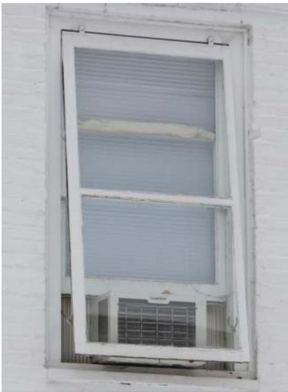
Figure 4.68 Window air conditioner prevents storm window from closing.
