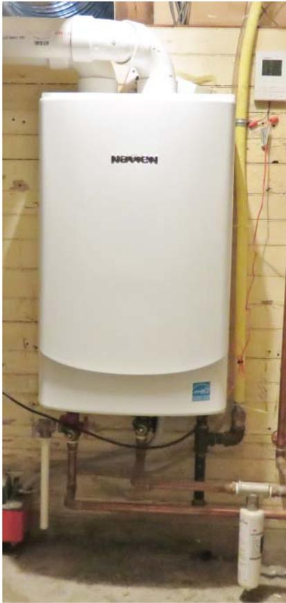
**Figure 12.7** Instantaneous water heater—note plastic vent and combustion air intake pipes (top), indicating a high-efficiency water heater.
