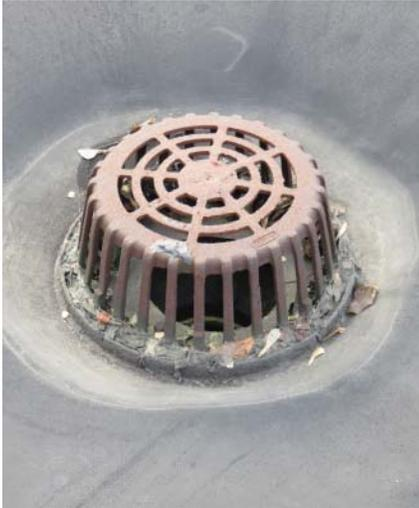
**Figure 4.20** Roof drain on flat roof, to which roof insulation is used to provide pitch for drainage.
