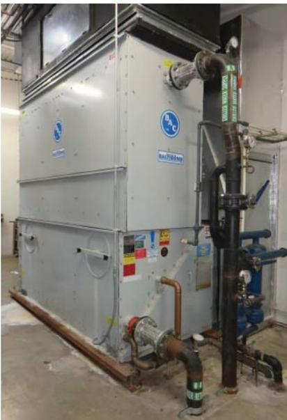
Figure 7.35 Cooling tower located indoors.
