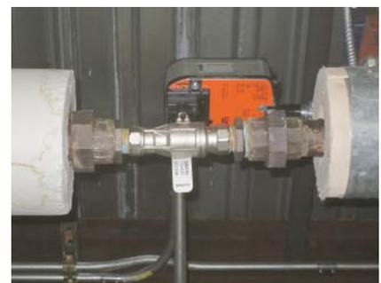
**Figure 11.15** Motorized valve.
