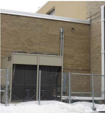
**Figure 7.13** Large commercial split system outdoor unit (condensing unit).
