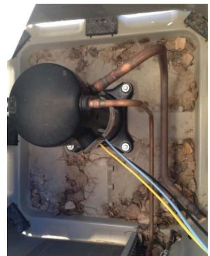
**Figure 10.2** Cooling-only outdoor unit (no reversing valve).
