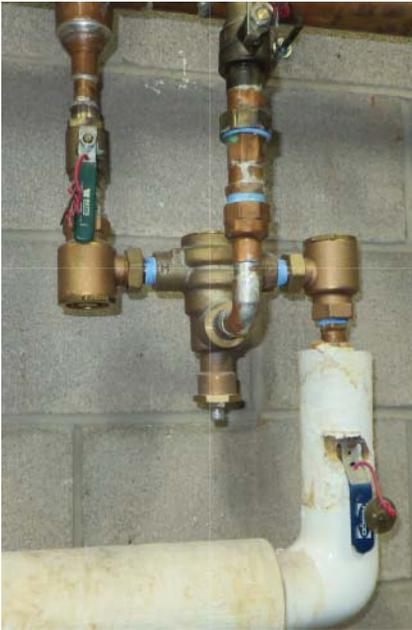
**Figure 12.11** Mixing valve—hot water enters from left (marked H), cold water enters from right (marked C), mixed water leaves at bottom.
