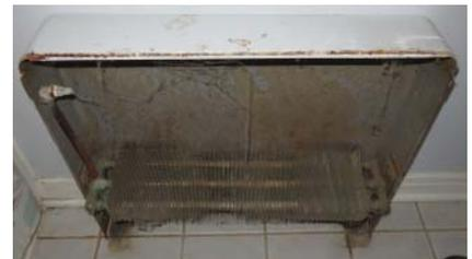
Figure 6.9 Cabinet fin tube radiator (cover removed).
