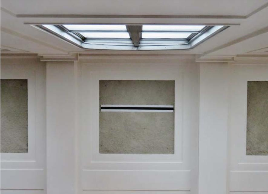
Figure 10.6 Linear diffuser.
