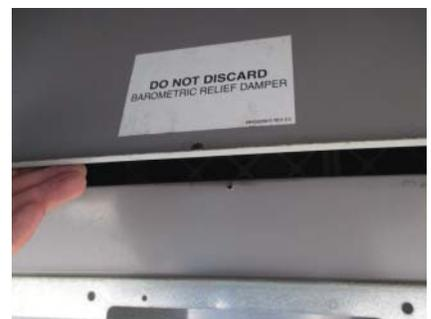
Figure 9.6 Relief damper built into packaged heating/cooling unit.
