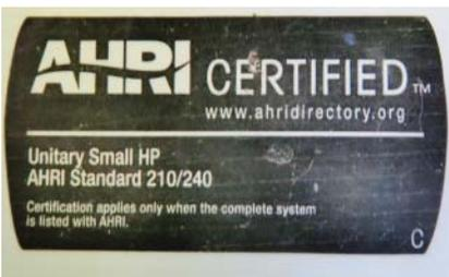
**Figure 10.10** AHRI label, which indicates the equipment is newer than 2007.
