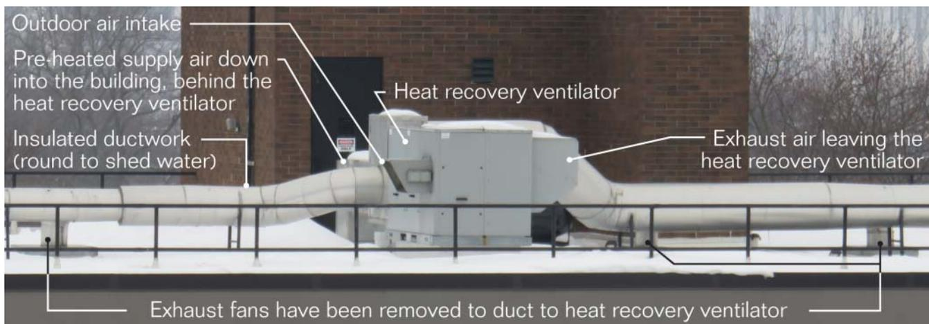
**Figure 9.20** Retrofit heat recovery ventilator.
