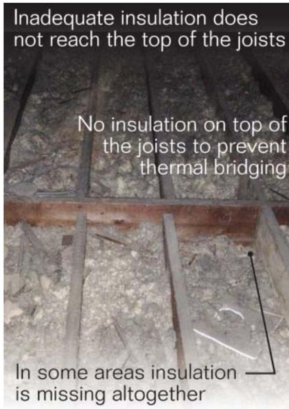
**Figure 4.15** Attic insulation deficiencies.
