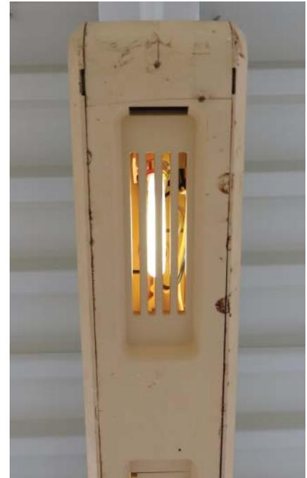
**Figure 5.40** Examining the bottom of an exit light to identify the lamp type.
