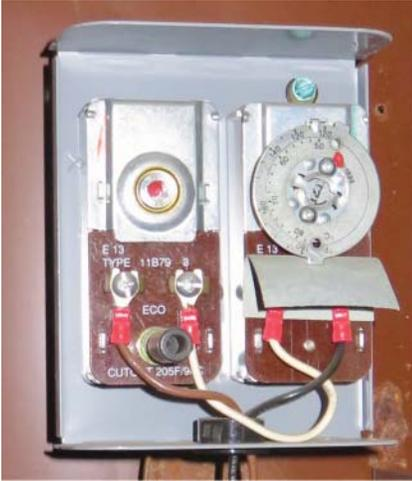
**Figure 12.10** Commercial water heater temperature control.
