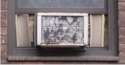
Figure 7.7 Fin damage.
