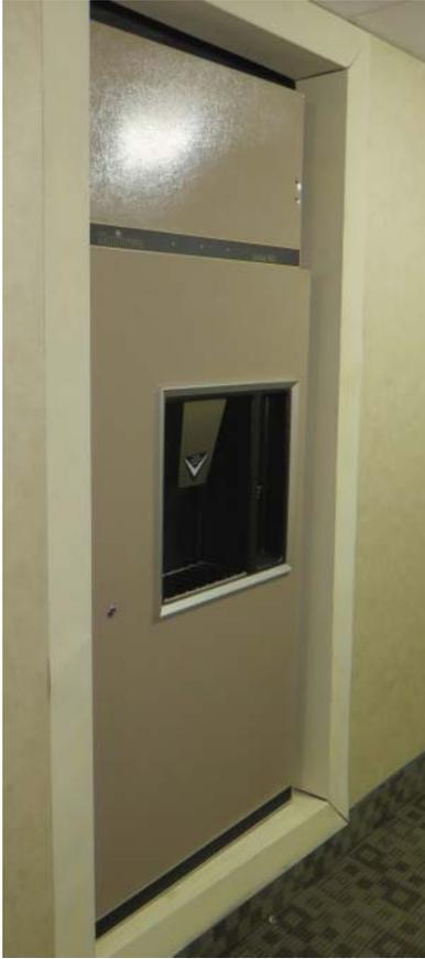
**Figure 13.9** Ice maker with insufficient clearance in a hotel corridor.
