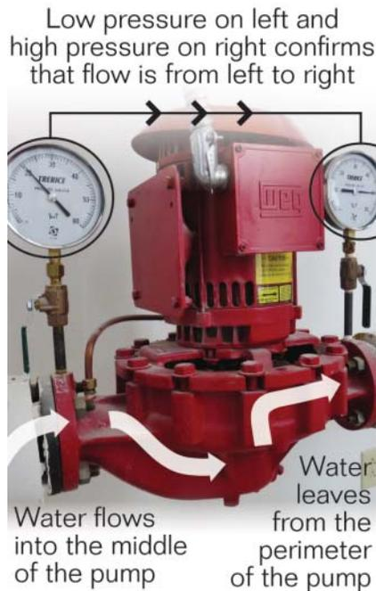
Figure 8.35 Pump flow direction.
