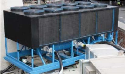
Figure 7.33 Air-cooled chiller.
