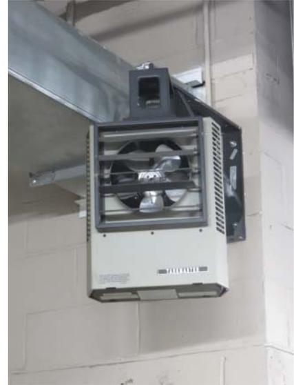
Figure 6.21 Electric unit heater.
