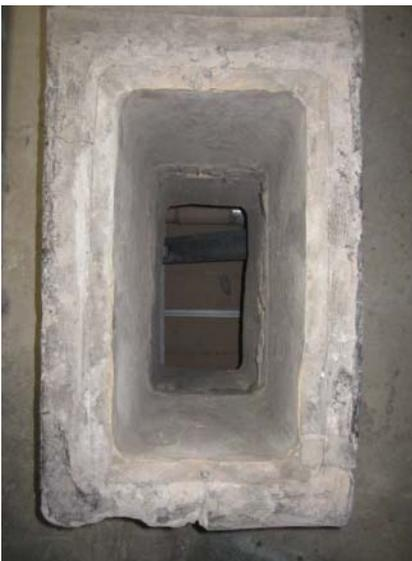
Figure 8.11 Masonry duct shaft, not capped, inadvertently open to ceiling plenum below.
