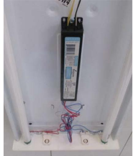
Figure 5.3 Fluorescent fixture ballast.
