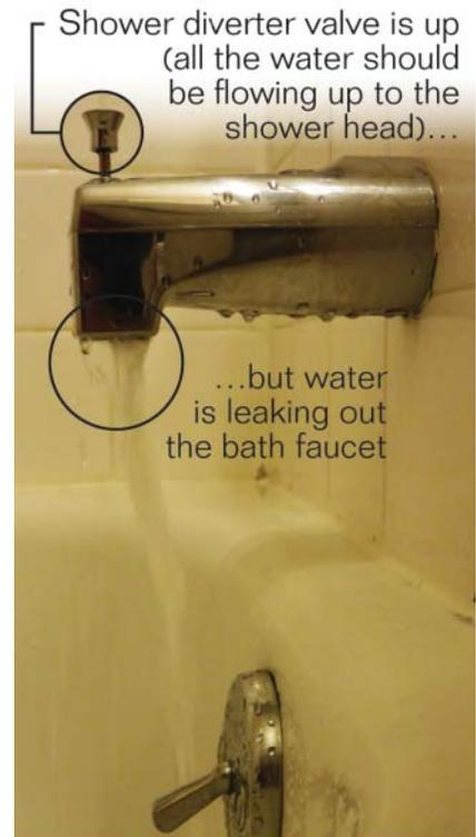
Figure 12.34 Leaking shower diverter.
