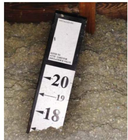
**Figure 4.19** Insulation depth marker.
