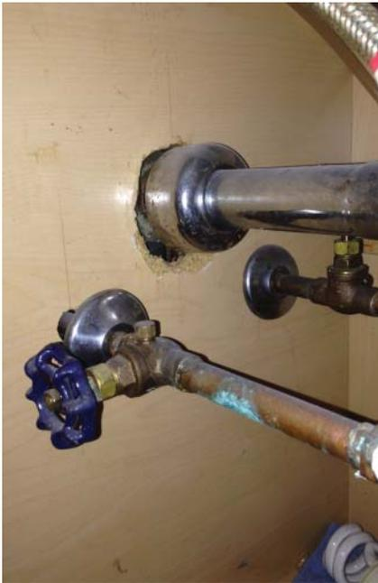
**Figure 4.59** Unsealed pipe penetrations—one escutcheon is not large enough to cover a pipe penetration hole, another escutcheon is loose and not sealed.
