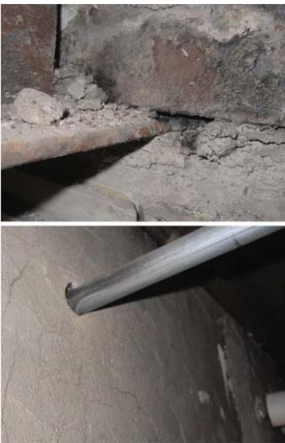
**Figure 9.14** Air leakage through structural, electrical, and piping penetrations into chases.
