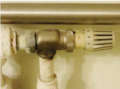
Figure 11.3 Thermostatic radiator valve.
