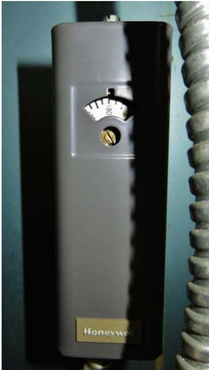
**Figure 6.6** Boiler-mounted water temperature control, or aquastat, with a fixed supply water set point of 180 F.
