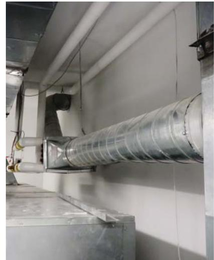
Figure 8.1 Spiral duct.
