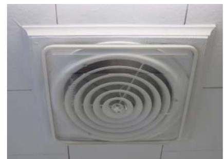
**Figure 4.75** Diffuser cover on a cooling-only forced air system, fastened with a tension fastener in the center of the diffuser, prevents infiltration during heating season.
