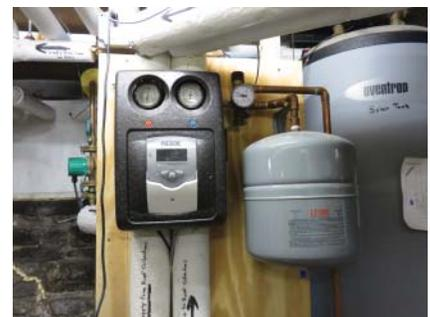
Figure 15.1 Solar thermal components.
