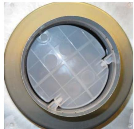
**Figure 4.66** Leaky backdraft damper in an exhaust fan.
