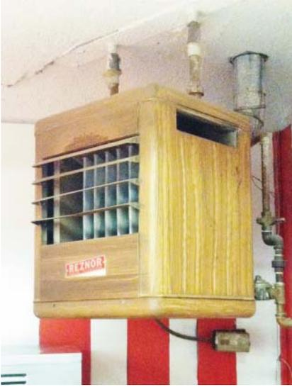
**Figure 6.19** Gas-fired suspended unit heater.
