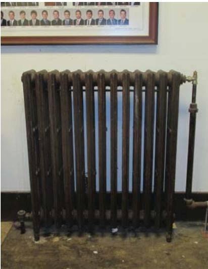
**Figure 6.15** Cast iron steam radiator, with pipe connection across the top—can be converted to hot water.
