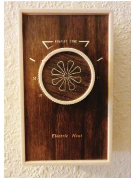
Figure 11.8 Line voltage thermostat.
