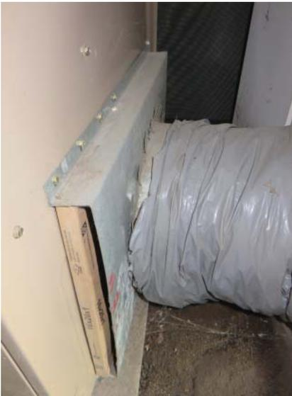
**Figure 6.20** Poorly sealed filter housing.
