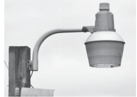
Figure 5.6 Mercury vapor light fixture.
