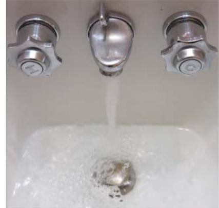
**Figure 12.16** High faucet flow over 2 GPM typically will fill a sink even if the drain plug is open.
