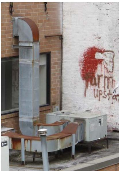
Figure 8.5 Corrosion on outdoor ductwork.
