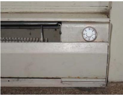
Figure 11.2 Equipment-mounted mechanical thermostat.
