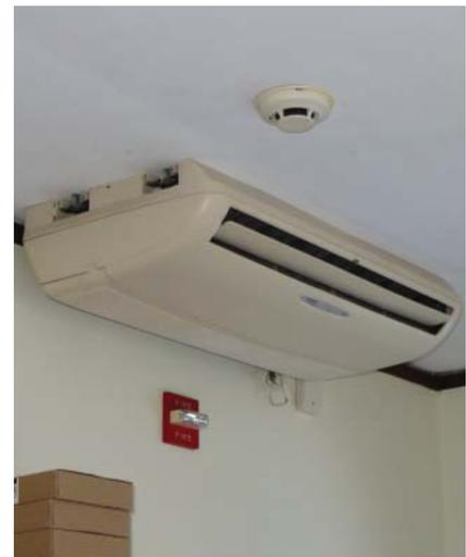
**Figure 7.16** Ceiling surface-mounted ductless fan coil.
