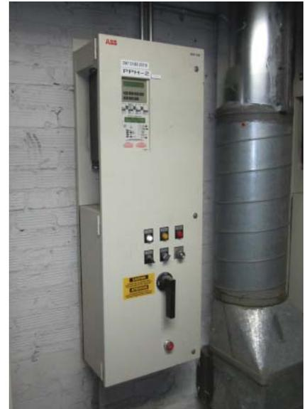
Figure 16.4 Variable-frequency drive.
