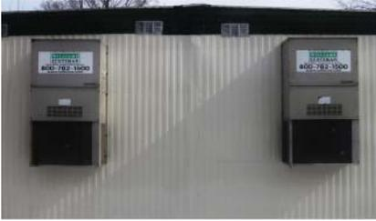
**Figure 7.27** Through-wall single-package units on a temporary classroom.
