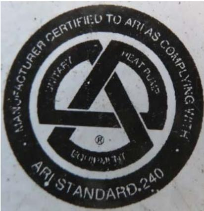
**Figure 10.9** ARI label, which indicates the equipment is older than 2007.
