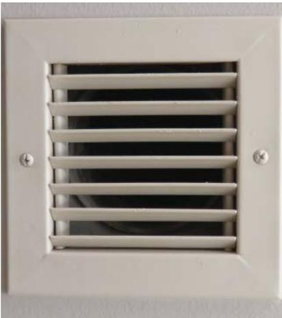
**Figure 9.9** Bathroom exhaust grille.
