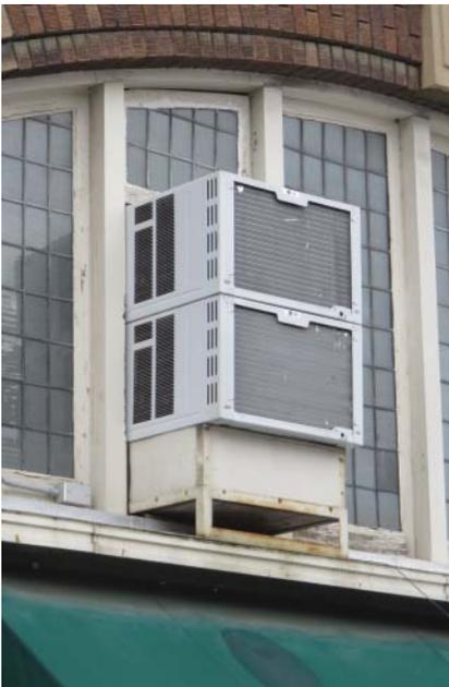
Figure 7.3 Room air conditioners are used in a wide variety of commercial building applications.
