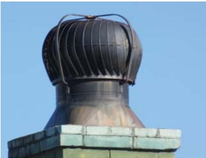
**Figure 9.8** Turbine ventilator.
