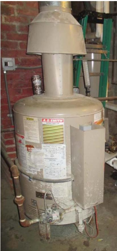
**Figure 12.4** Natural gas water heater.
