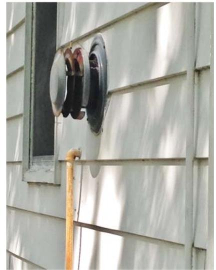
Figure 6.16 Wall-mounted vented gas room heater. It is identifiable as gas fired by the gas pipe on the outside wall, and as vented by the vent on the outside wall.
