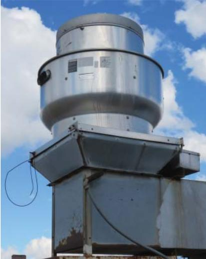
Figure 9.1 Upblast exhaust fan.
