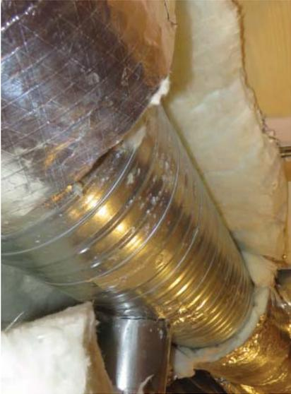
Figure 8.9 Detached duct insulation.
