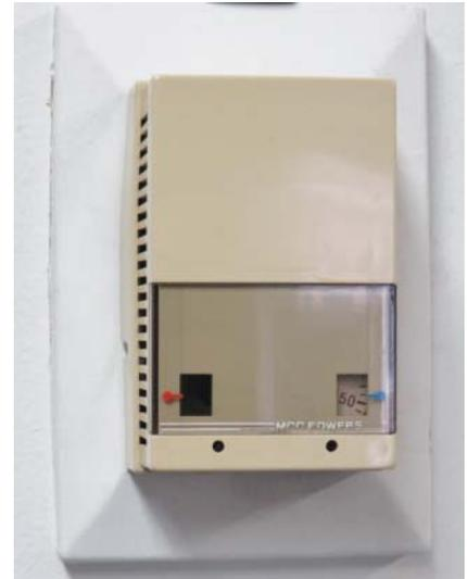
**Figure 11.13** Temperature sensor with limited local control.
