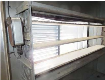
**Figure 11.17** Outdoor air damper and motor actuator.
