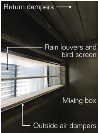
**Figure 9.13** Outside air intake, seen from inside an air handler.
