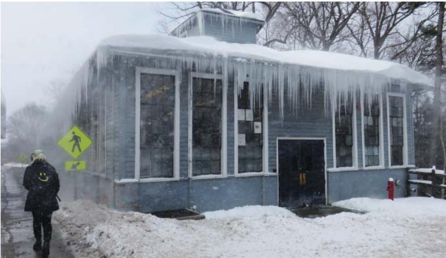
**Figure 3.9** Ice dams as an indicator of catastrophic heat loss.
