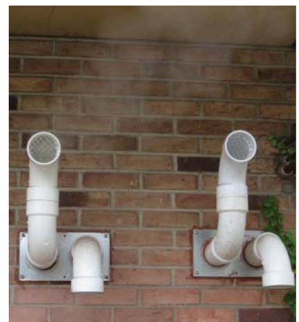
Figure 6.5 Plastic vent piping (upper pipes are combustion exhaust, lower pipes are combustion air intake).
