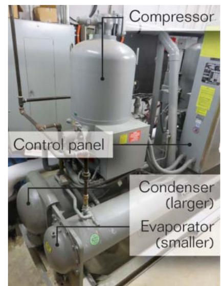
Figure 7.32 Water-cooled chiller.
