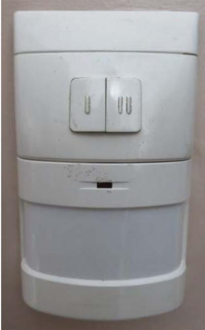
**Figure 5.27** Motion sensor with two levels of control.
