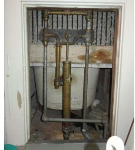
**Figure 4.69** Infiltration sites below/around bathtub framing.
