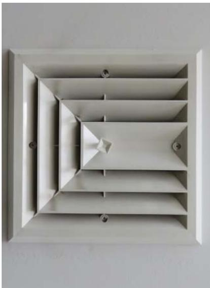
**Figure 10.5** Supply diffuser.
