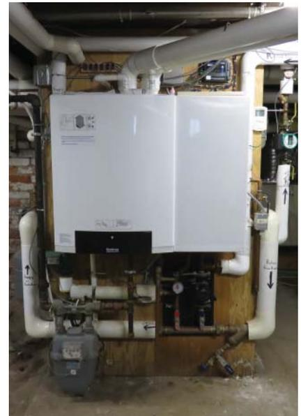
Figure 6.4 Condensing wall-hung boiler.
