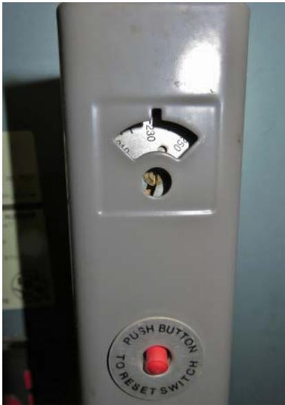
**Figure 6.7** Boiler-mounted water temperature high-limit safety switch.
