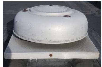
Figure 9.5 Gravity ventilator.
