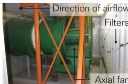
Figure 8.24 Air handler—fan section.
