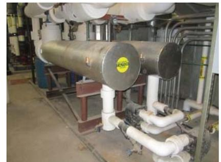
Figure 6.13 Hot water generator (steam-to-water heat exchanger).
