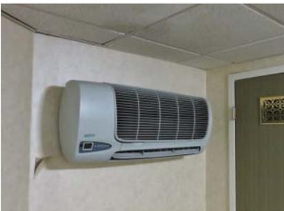
**Figure 7.14** Wall-mounted ductless indoor unit.
