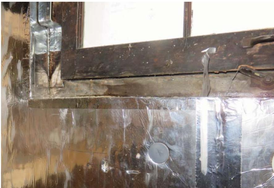
Figure 4.24 Rigid insulation directly fastened to a basement wall, foil-faced to provide required fire resistance.
