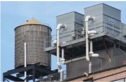
Figure 7.34 Roof-mounted cooling tower.
