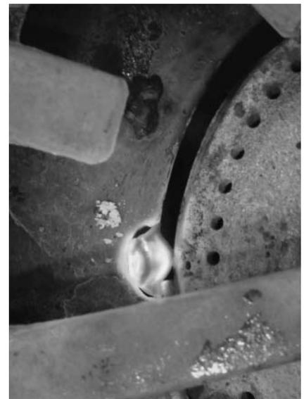
**Figure 14.1** Standing pilot on a commercial stove burner.
