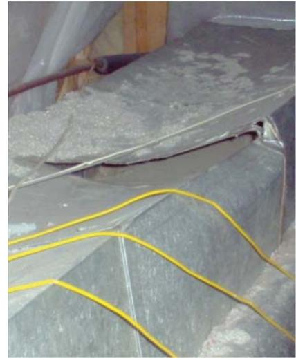
Figure 8.12 Catastrophic duct failure.
