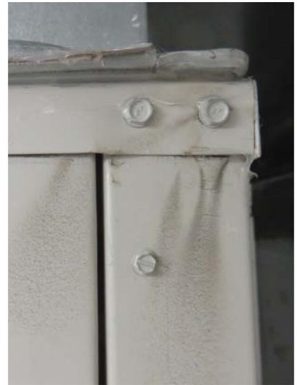
Figure 8.18 Dust or dirt is a sign of air leakage.
