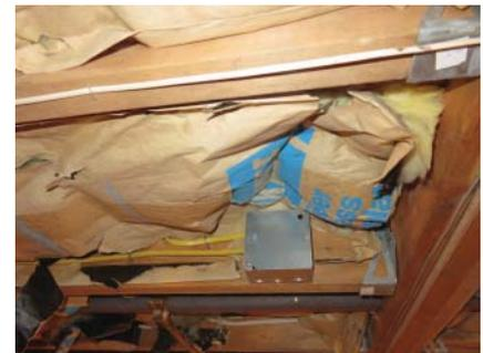
Figure 4.8 Compressed insulation.
