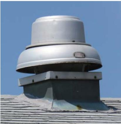
Figure 9.2 Downblast exhaust fan.
