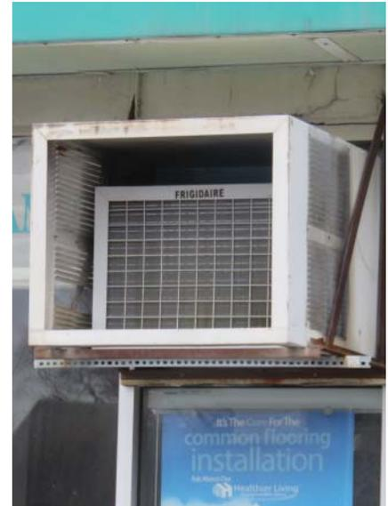
**Figure 4.64** Room air conditioner in ill-fitting sleeve
