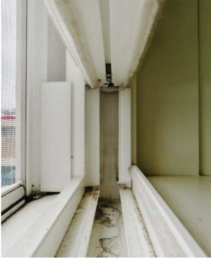
**Figure 4.76** Weather-stripping prevents infiltration at four locations on a window sash—on the front and back edges, and in two locations below the sash.
