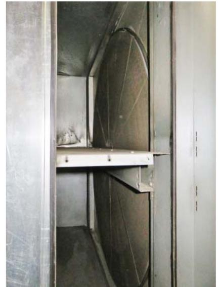
**Figure 9.18** Rotating-wheel heat recovery ventilator.
