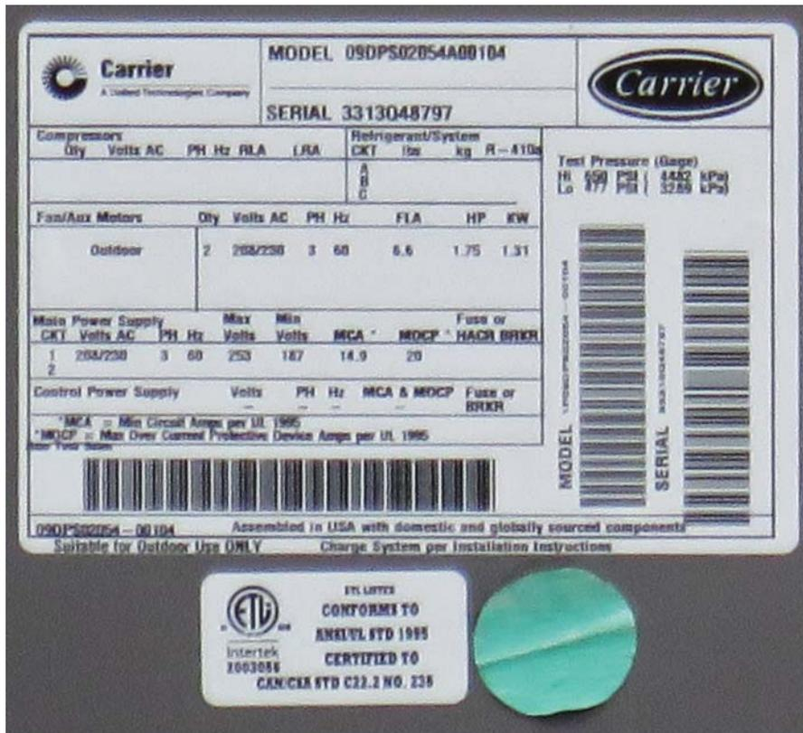
Figure 3.7 Photograph of air conditioning nameplate on a rooftop, taken standing at ground level, 66 feet away, 30x optical zoom with 120x digital zoom.
