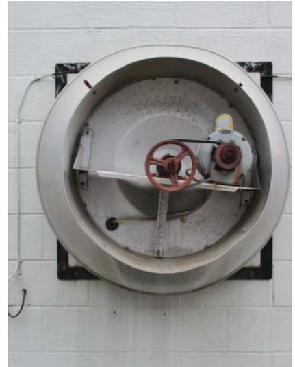
Figure 9.4 Belt-driven exhaust fan.
