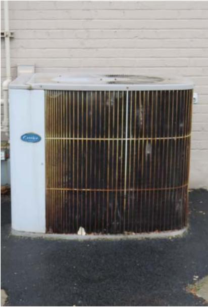
**Figure 10.8** Significant rust indicates a unit that is likely over 20 years old.
