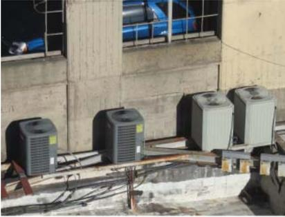
**Figure 7.12** Residential split system outdoor units (condensing units) used in commercial buildings.
