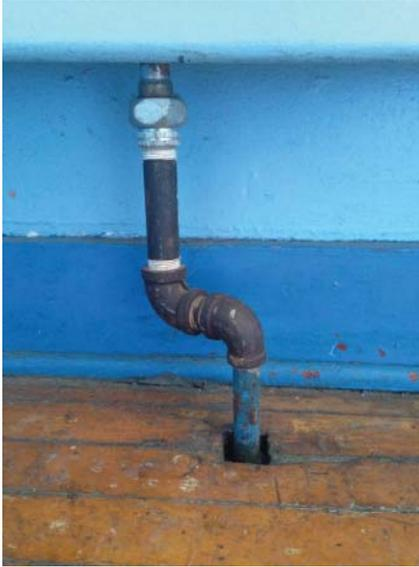
Figure 4.62 Unsealed pipe penetration.
