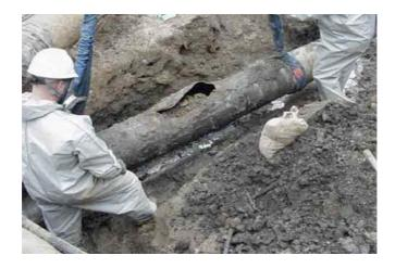
Figure 1.1 Actual rupture in the pipeline
