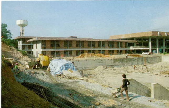
Kiri: Pembinaan giat dijalankan. Left: Construction in progress.
