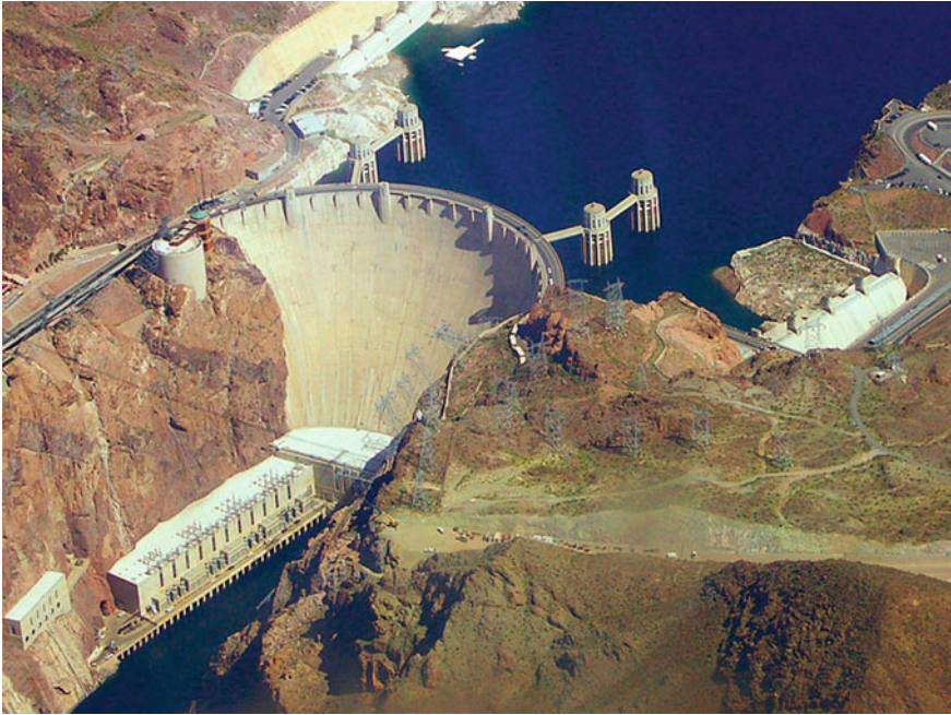
Fig. 4.6 The Hoover Dam in the USA is a large conventional dammed-hydro facility, with an installed capacity of 2080 MW (Source http://en.wikipedia.org/wiki/Hoover_Dam )
