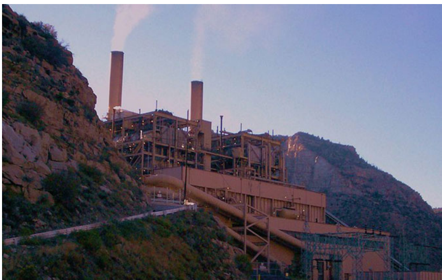
Fig. 2.6 A coal-fired power plant in Utah, USA ( Source http://en.wikipedia.org/wiki/Fossil-fuel_power_station )
