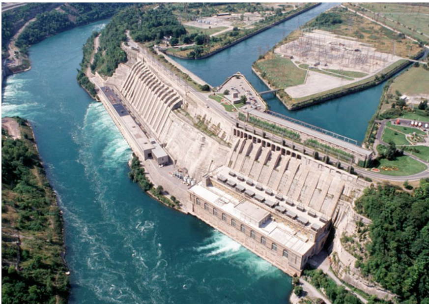
Fig. 6.5 Sir Adam Beck generating complex acknowledgement Ontario power generation. Source https://en.wikipedia.org/wiki/Wind_power
