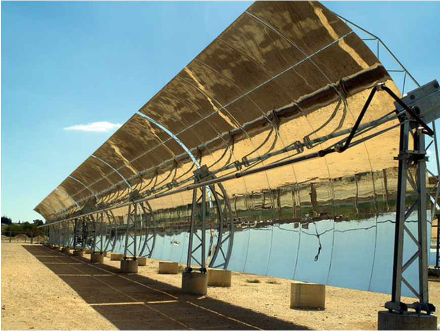
Fig. 4.3 Array of parabolic troughs at the National Solar Energy Centre in Israel (Source http://en.wikipedia.org/wiki/Parabolic_trough )
