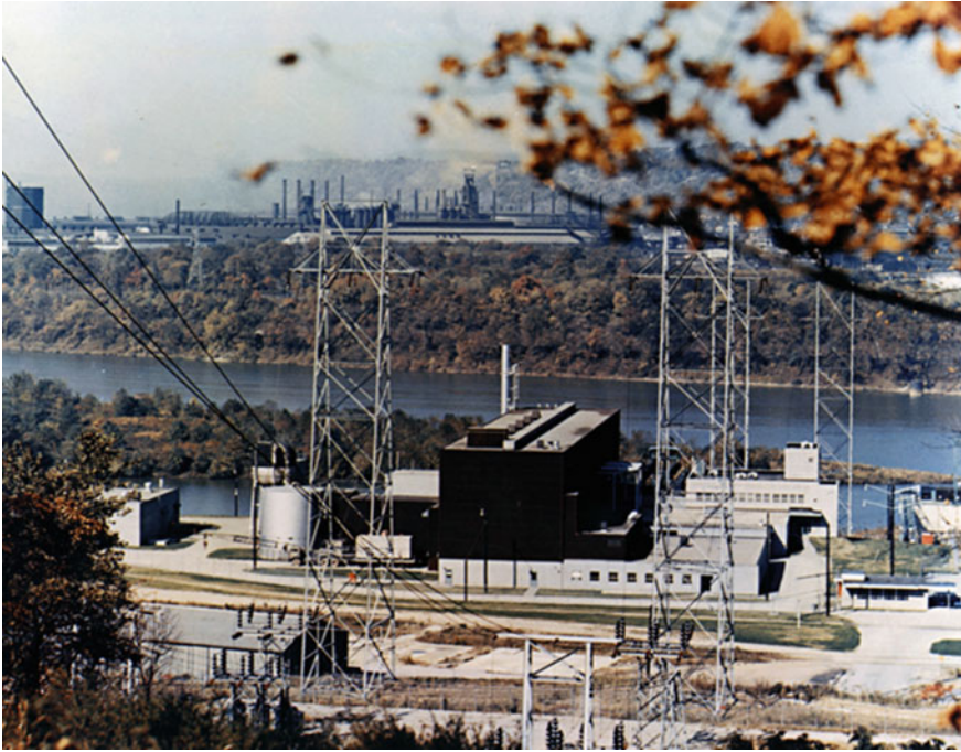
Fig. 4.12 The Shippingport Atomic Power Station, Pennsylvania, USA (Source http://en.wikipedia.org/wiki/Nuclear_power )
