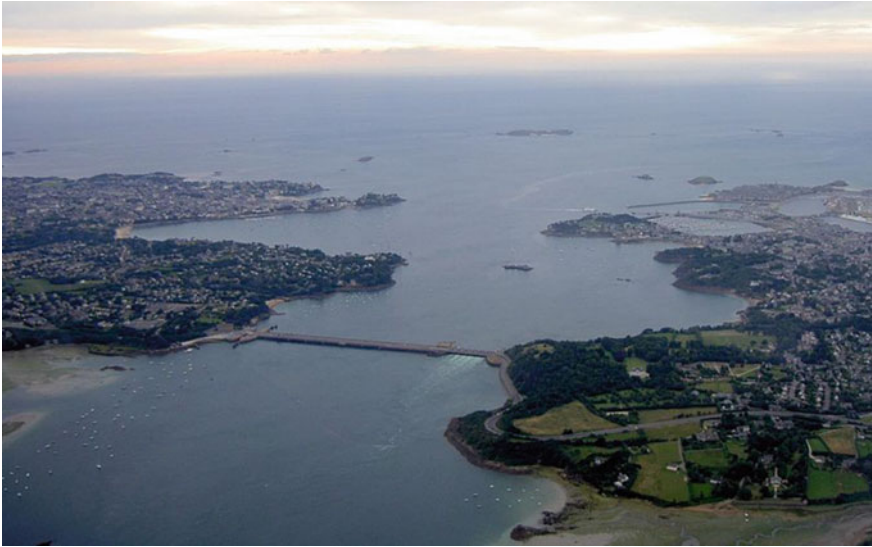
Fig. 4.7 Aerial view of the Rance Tidal Barrier and generating station (Source http://en.wikipedia.org/wiki/Rance_Tidal_Power_Station )
